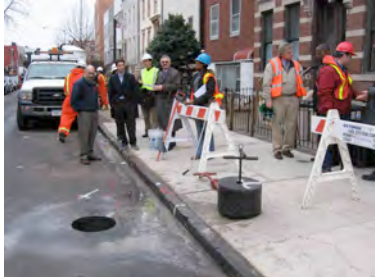
3. 13-inch asphalt core
