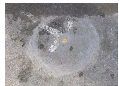
10. Reinstated core – almost invisible
