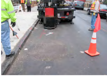
1. Coring unit with conventional repair in foreground
