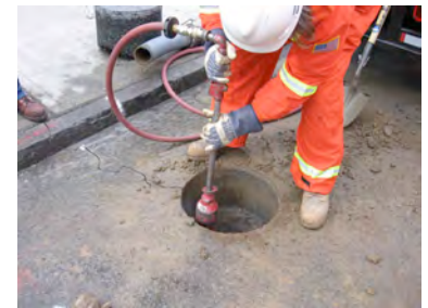
7. Compaction (note wire from soil compaction supervisor)
