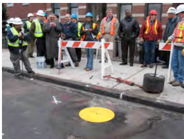
4. Temporary road plate
