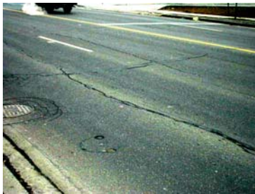
Figure 5. Pavement core reinstated in bus lane with Utilibond in 1995 still in perfect condition seven years later in 2002.
