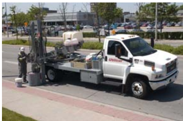
Figure 1. The Utilicor coring unit operates through a complete 270° arc, allowing the truck to be positioned on the shoulder or off the traveled surface to minimize traffic disruption.
