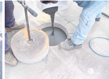
Utilibond poured into hole
