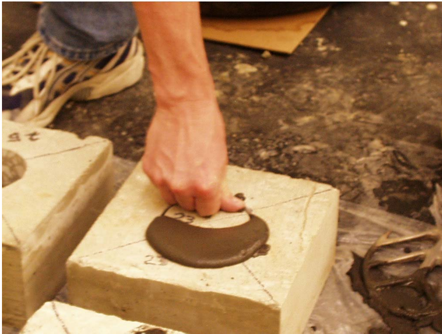
Photo 4. Reinstatement of core
