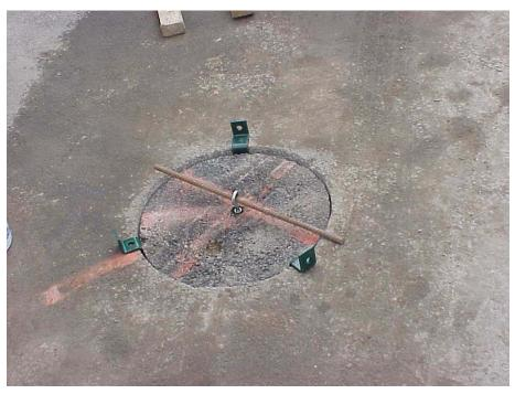
Figure 38. Pre-marking and anchoring the core
