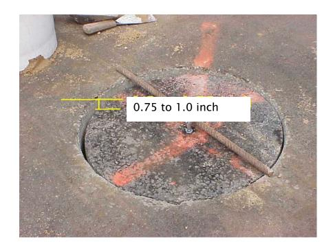
Figure 40. A uniform grout bed of 0.5-0.75 inch was set by placing the core on top of backfill before adding the grout.
