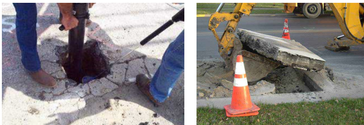
Figures 8 and 9. Damage around the utility cut caused by jackhammers and backhoes
