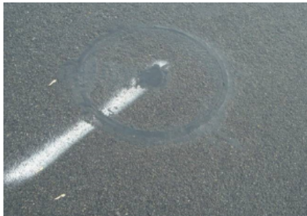
Figure 2. Keyhole pavement restoration
